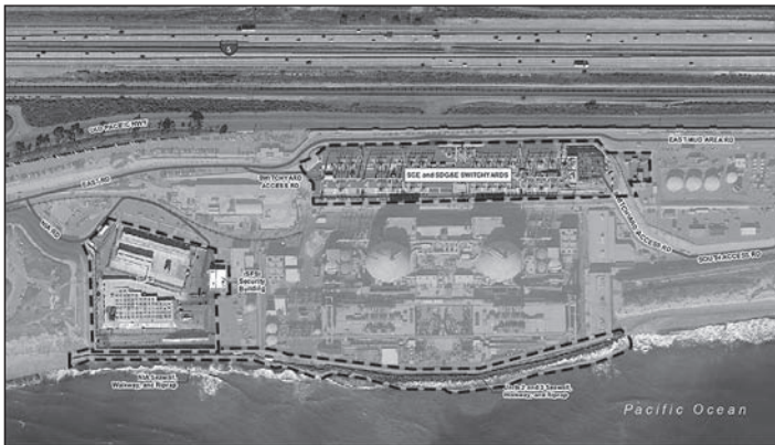
Aerial view of the SONGS site: After the demolition of units 2 and 3 buildings, the areas remaining are outlined by dotted black lines. The “interim” storage area (ISFSI) at the left (north) of the site and the power substation switchyards (closer to I-5 on the east side of the site) will remain, and the rest of the site will be cleared to 3 feet below grade. Picture from the CCC staff report.
