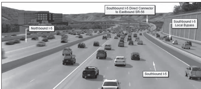
Drivers traveling southbound on I-5 would exit via the SR-56 east ramp. Drivers exiting to Carmel Valley Road are on the right using the local bypass from Del Mar Heights Road.
