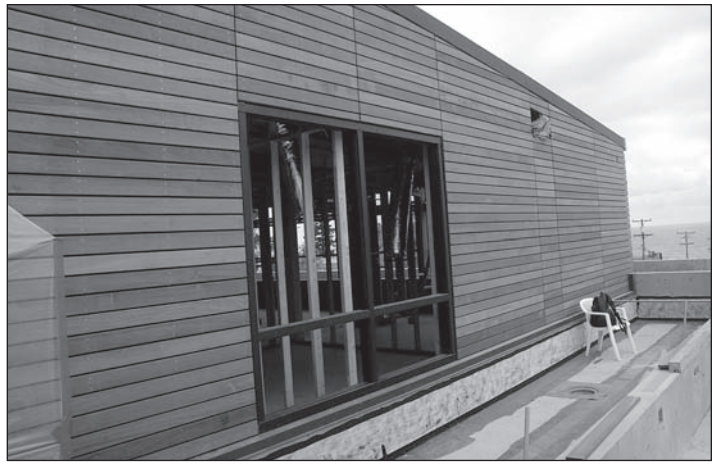
The view of the north wall of City Hall looking west shows the ipe wood siding. Ipe is a dense, renewable wood that is extremely durable, and is being used in many exposed elements to withstand the impacts of the coastal environment.
