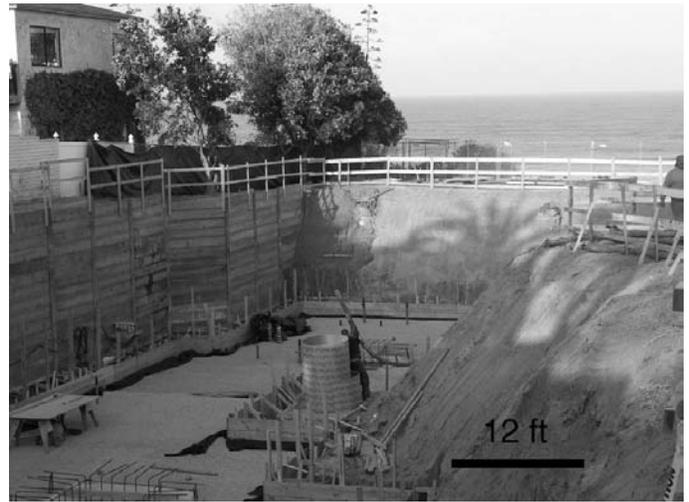
*Excavation for a house under construction on Ocean Avenue. The depth of the excavation is approximately 20 feet. Note pilings and shoring near neighboring property at the left (south) of picture. Picture courtesy of Art Olson.*
