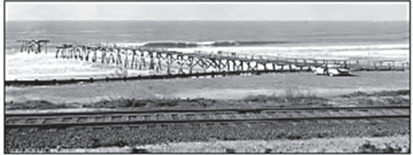
The pier in 1958. The pier was demolished by Navy frogmen in 1959 after severe damage in winter storms.
